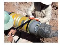
SIMPLE MARKING BAND SYSTEM MAKES REPAIRS VISIBLE TO IN-LINE INSPECTIONS
